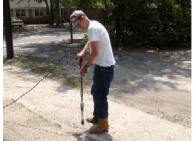
Harl Porter Pressure Washes the Driveway
